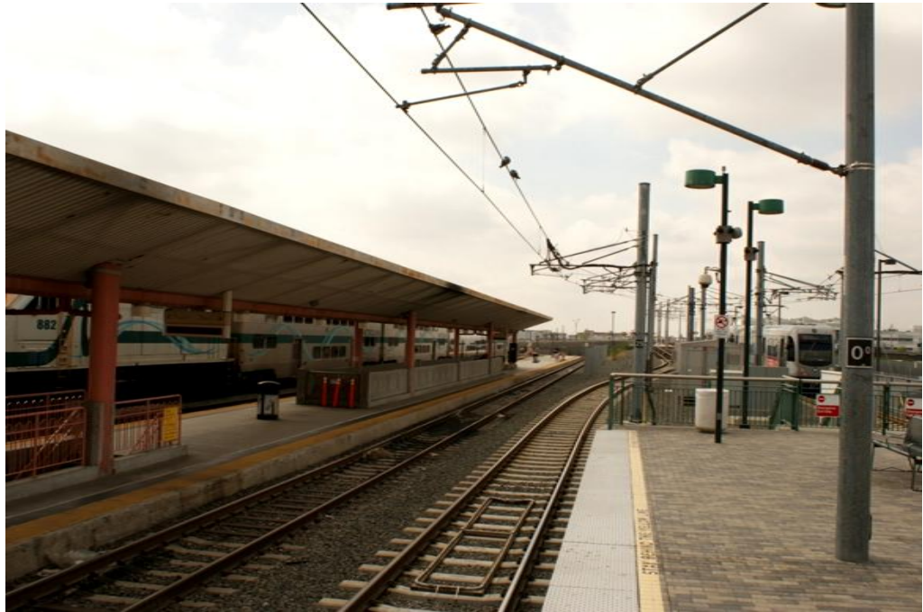
Station Union Station, Gold line – Photo Jean Leveugle
